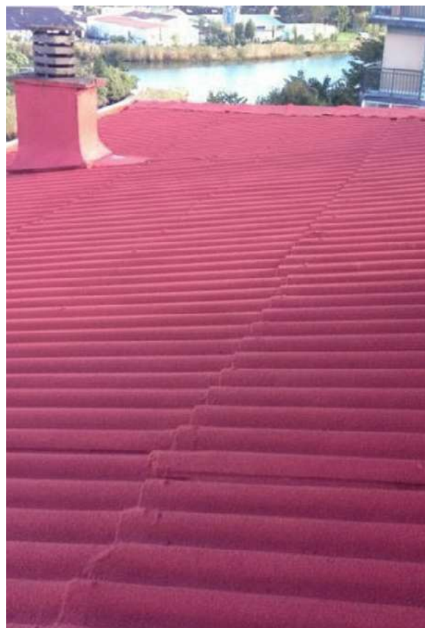
Roof after treatment with VIPEQ F10
